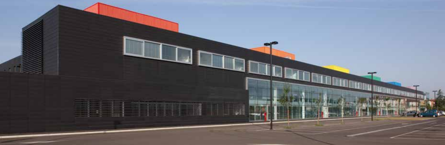
vista del lato nord est view of the north-east side
