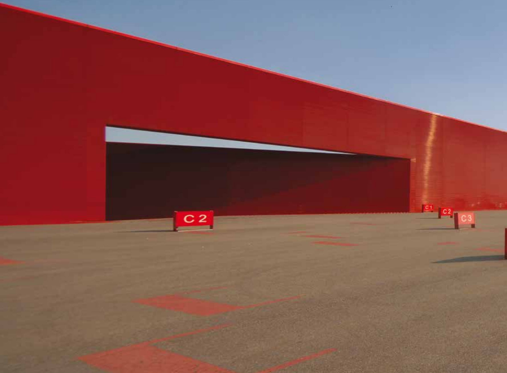
vista lato parcheggio/view from the parking lot
