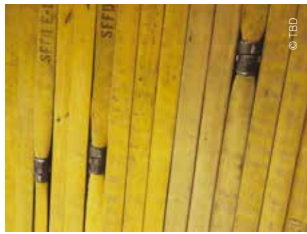
pompe antincendio rivestono una parete interna/salvaged fire hose as interior wall covering
